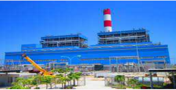
Vinh Tan thermal power plant Contractor: Posco E&C - KOREA
