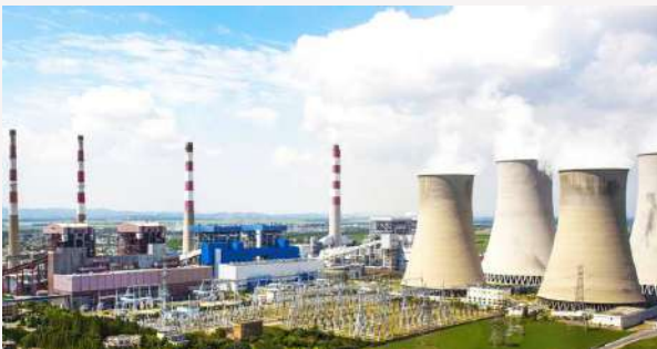
Nghi Sơn 2 thermal power plant - Thanh Hoa province Contractor: Doosan Heavy Industries - Korea
