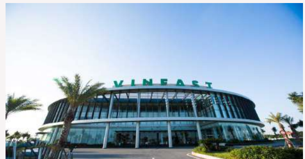
Vinfest Automobile factory Contractors: Cotecons, Unicons, Ricons - Vietnam
