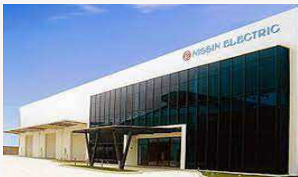
NISSIN Vietnam factory Contractor: Yurtec - Japan
