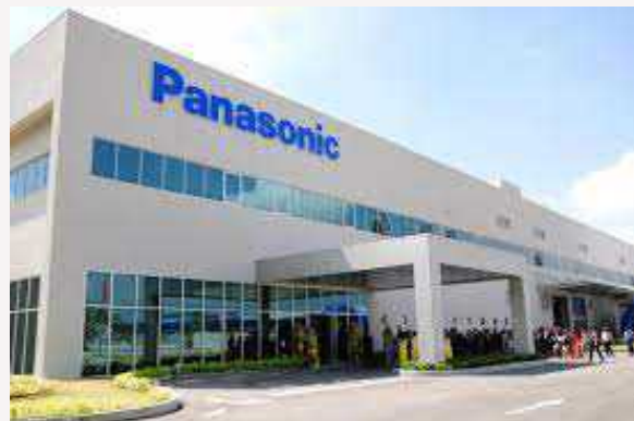
Panasonic Thanglong factory Contractor: Takisha - Japan
