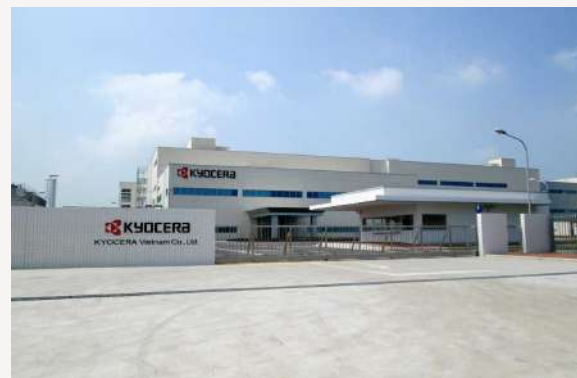
Kyocera factory Contractor: Kinden - Japan
