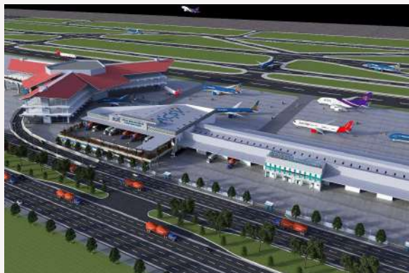
ASCV cargo station Noibai airport - Hanoi Contractor: Hawee - Vietnam
